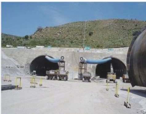
Figure 1: General view of the tunnel T4
