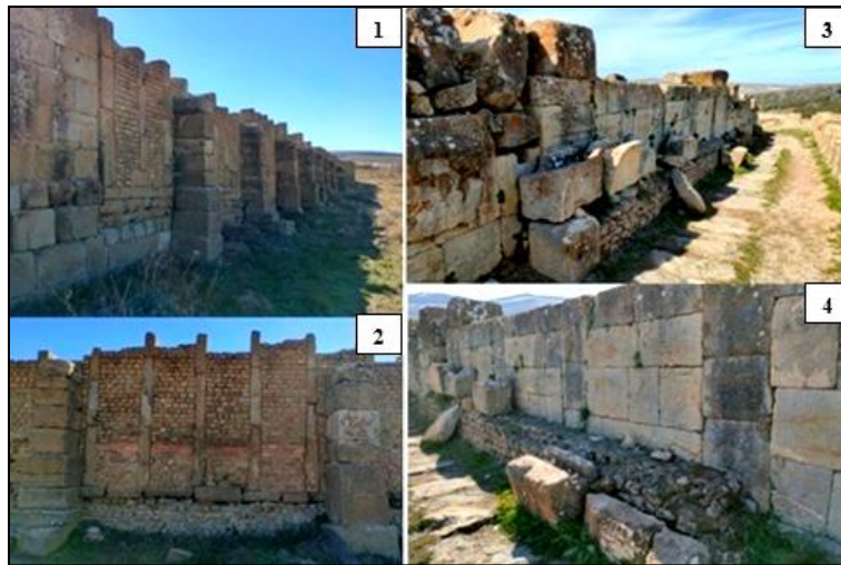
Figure 7: Buttresses (source: Author 2023). Numbers 1 & 2: External buttress pillars at Timgad, Numbers 3 & 4: Reinforcement wall at Djemila.
