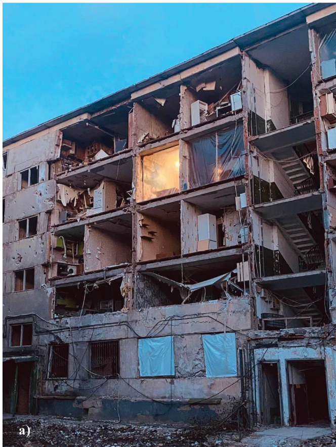
Fig. 1 Examples of partially destroyed large-panel buildings
