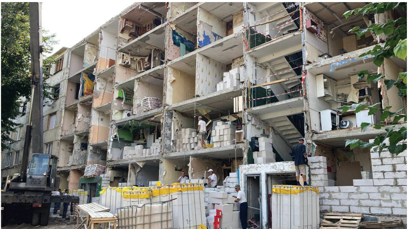
Fig. 5 The repair process of a large-panel building (sources: Information at https://cdn4.suspilne.media/images/resize/1040x1.78/680874f014cfd08.jpg )
