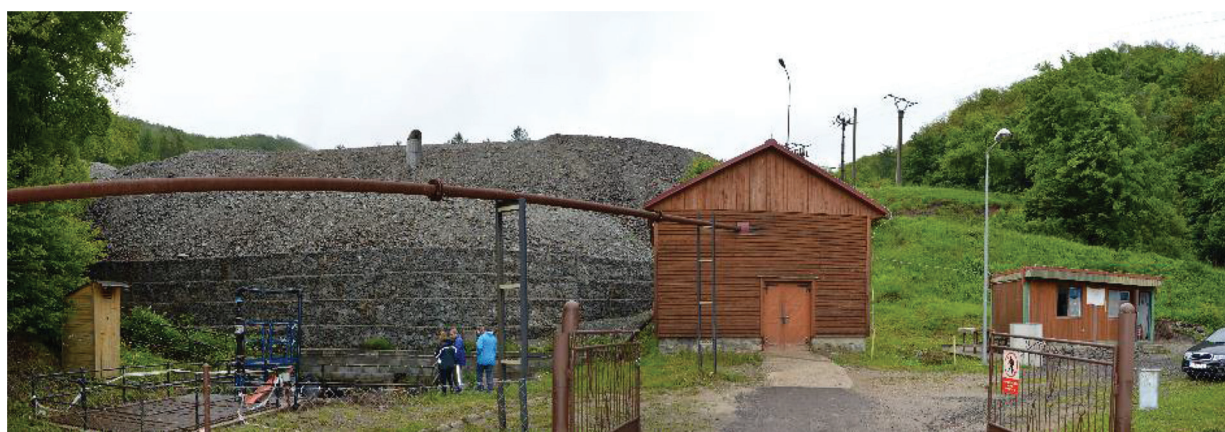
Fig. 3 Frontal view of the base dam of the tailings pond with a gabion wall
