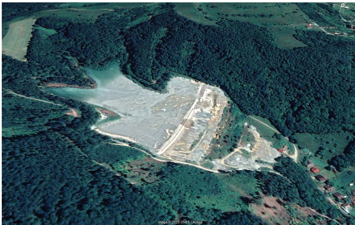
Fig. 1 The aerial view of the tailings pond
