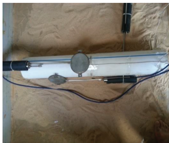
b. Pressure cell placed on the pipe surface.
