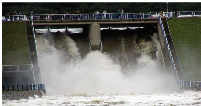
Fig. 9 The original spillway almost choked up during the flood in 2002 (VD-TBD, 2021)
