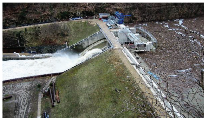
Fig. 10 Reconstructed spillway with steel traps during the flood in 2006 (VD-TBD, 2021)
