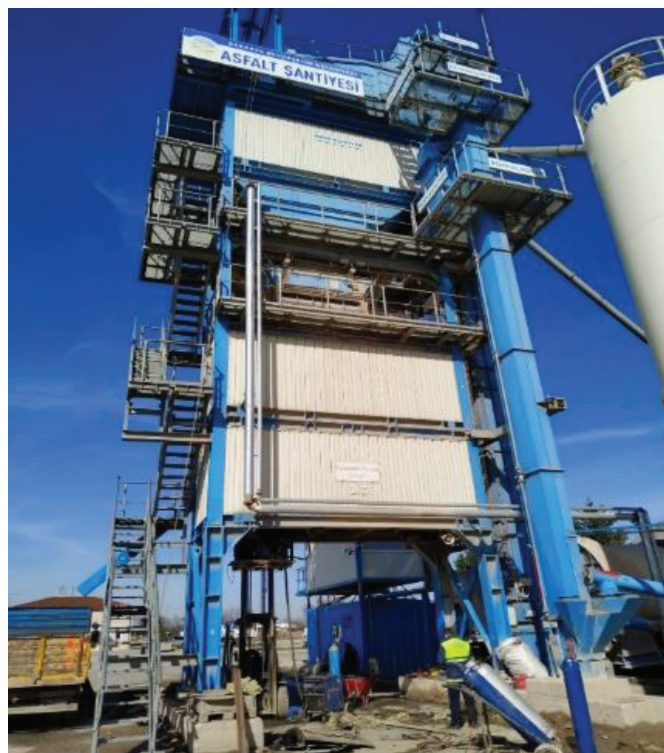
Fig. 10 ECO 4000 Benninghoven module plant
