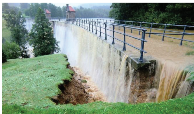
Fig. 12 Overtopping of the Mlýnice Dam during the flood in 2010 (VD-TBD, 2021)
