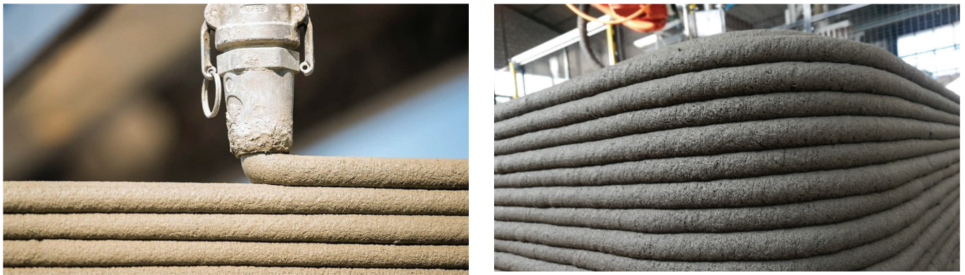
Fig. 1 Example of material and extruded construction using 3D concrete printing (Source: Kauppila I., 2021, CreaBeton Materiaux, 2019)
