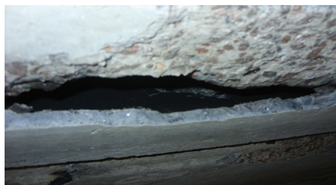
Fig. 2 Explosive layer-by-layer destruction of the protective layer of concrete on the side of the flames. The through cracks in the concrete bridges between the voids have opening widths of a = 11.5 and 21.5 mm, respectively
