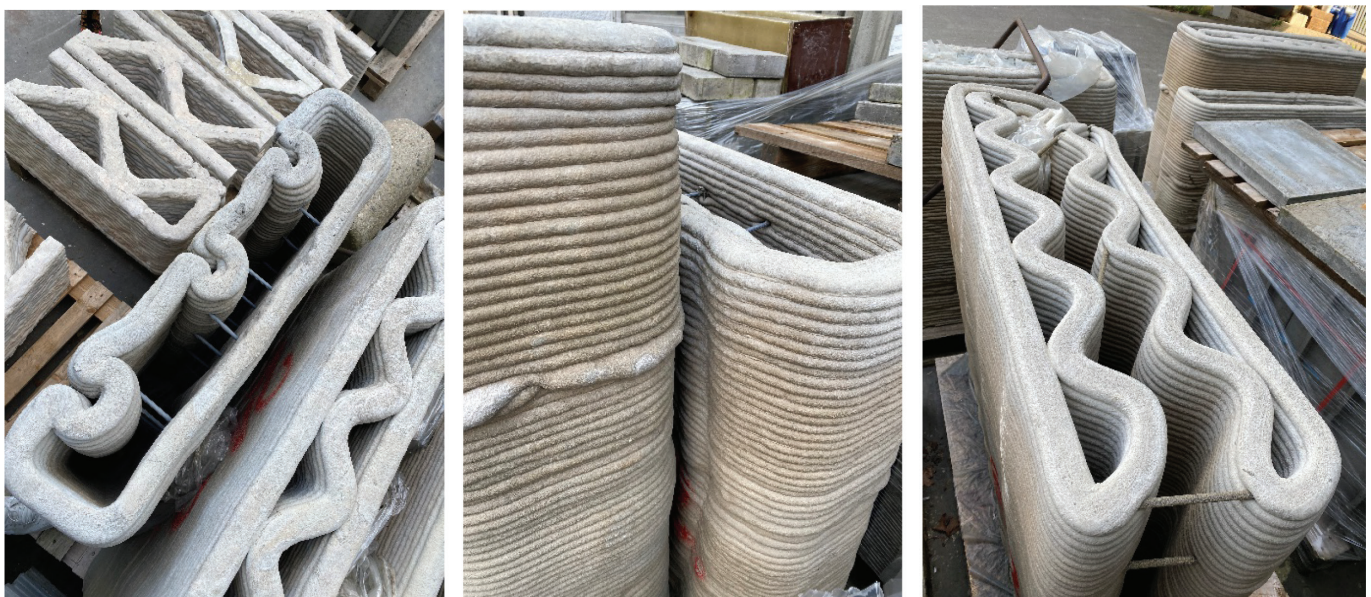
Fig. 7 Construction printed by a 3D printer at the Prague Technical University (Source: photos by the author: Uhlík, A. 2021)
