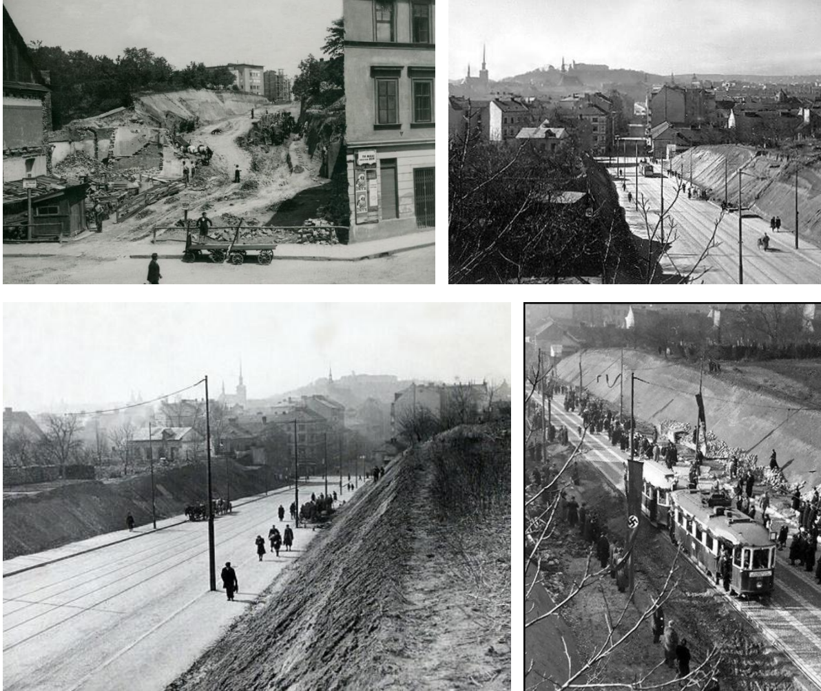
Fig.2 Historical photography of the newly created street, Demolition of the building and penetrating the block (top left), Newly paved and finished street (top right, bottom left), Nazi party celebrating first tram ride of the street (photographies provided by encyklopedie.brno.cz )
