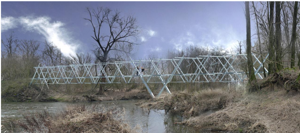
Fig.1: Tensegrity Footbridge / Petra Buganska
