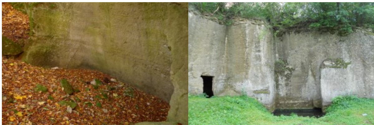
Fig. 8 The first step of the excavation of the underground chamber - the wall is modified into a "cell" in which the underground chamber began to be gradually mined at the foot-wall. The stone quarry of Chtelnica (on the left) and the stone quarry Krupina (on the right) (photo by P. Hronček)
