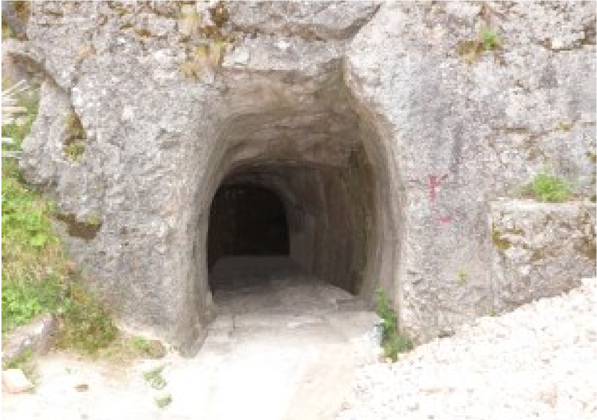
Fig. 6 Extracted underground (access tunnel) on Lednice Castle. This medieval tunnel is the oldest on the territory of Slovakia (photo by P. Hronček)
