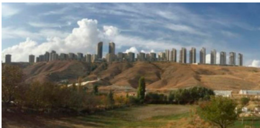
Figure 3 The constructions rising on the valley floor, slopes and upper parts of the valley destroy all ecological functions of the valley in the form of concrete walls (2019)
