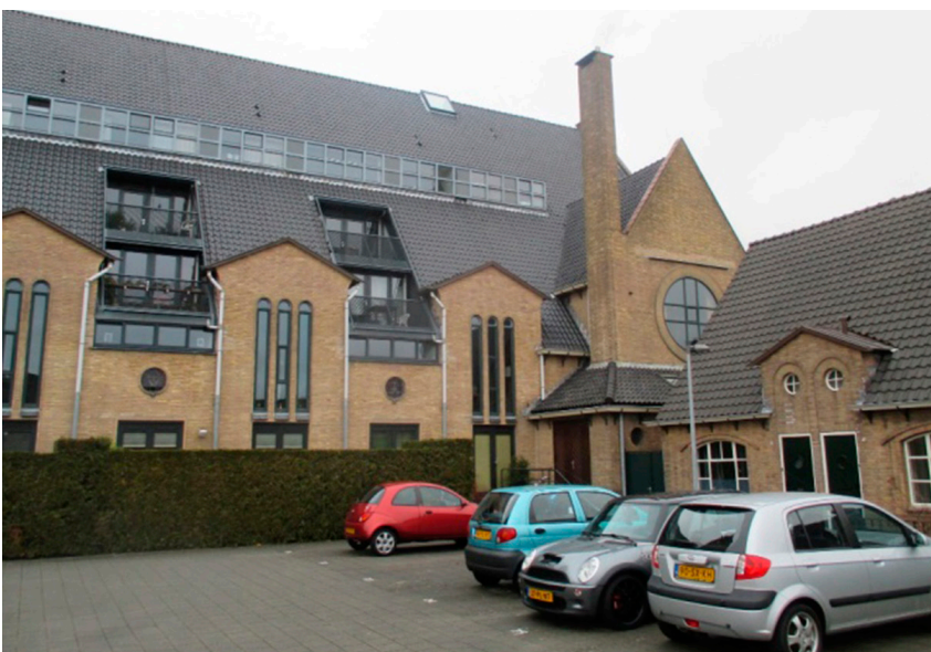
Figure 4 The re-utilisation of the St. Josephskerk (Hilversum) with apartments required structural changes of the façade necessary to provide sufficient lightning and ventilation of the apartments and open spaces (case 35) Photo: authors
