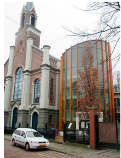
Figure 2 Creating an additional entrance of the Remonstrantse Kerk (Groningen) was necessary to provide a functional access to the office wing, used by the 'Stichting Oude Groninger Kerken' (case 19) Photo: authors
