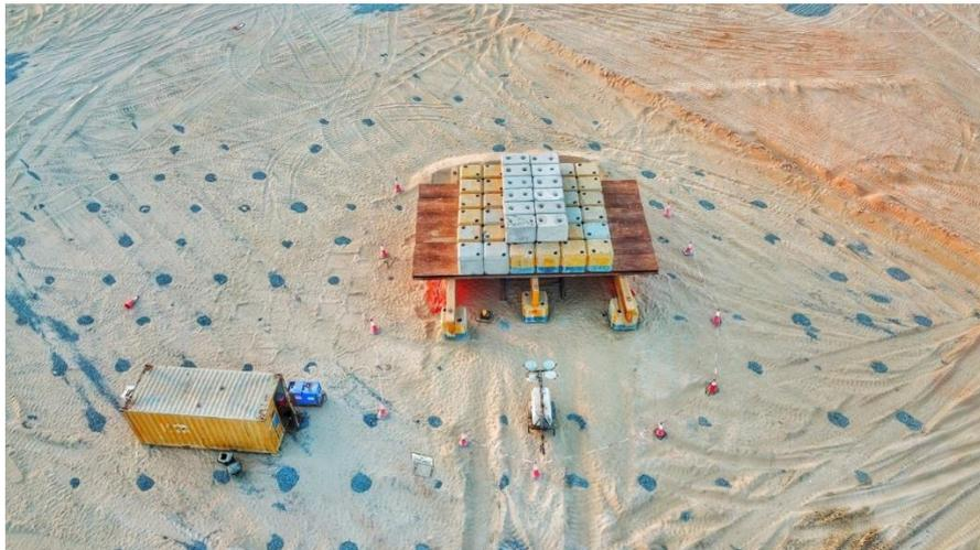
Figure 11: ZLT on the ground treated by stone columns
