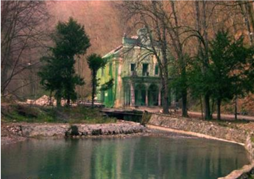
Figure 14: Old thermal water treatment base
