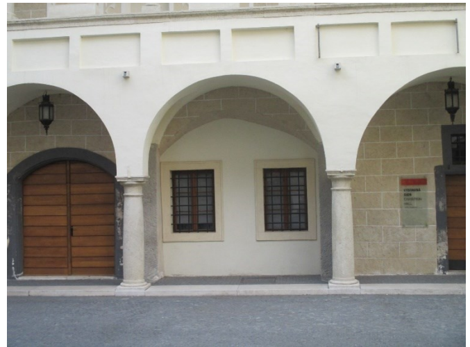
Fig. 7. The southern facade in the courtyard – middle part of the ground floor. (Photo: Author, 2020)
