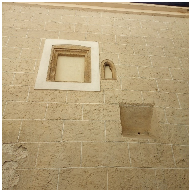
Fig. 21. Detail of the middle part in Kostolná Street with older medieval pointed window, younger medieval rectangular window and ventilation hole. Presented as niches. The surface is decorated with medieval network. (Photo: Author, 2023)
