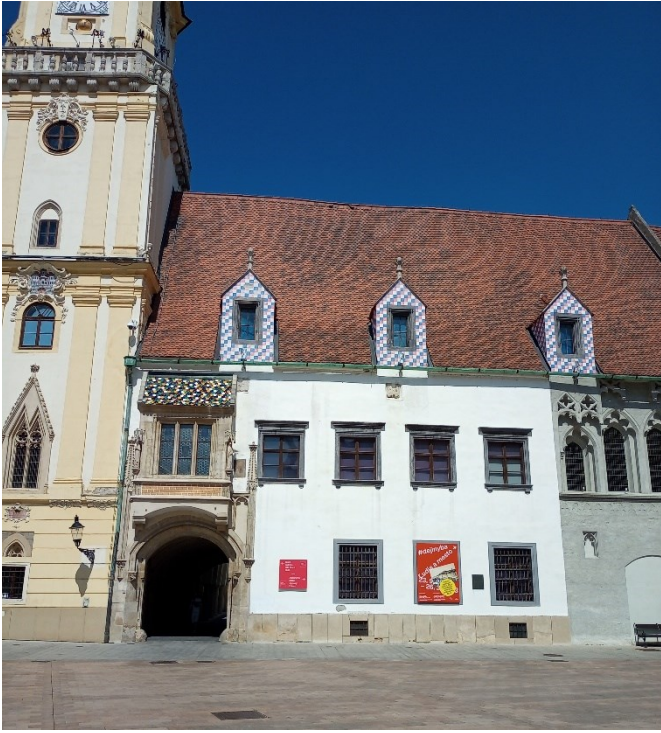
Fig. 10. Detail of the northern part – next to the tower is a part with the late Gothic portal and oriel above it. (Photo: Author, 2023)
