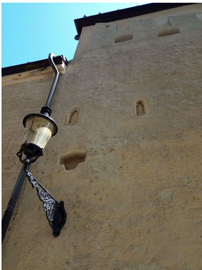
Fig. 19. The facade in the Kostolná Street – part with medieval windows, (niche), shooting range (embrasure) and battlements. Reconstructed medieval plaster. (Photo: Author, 2023)
