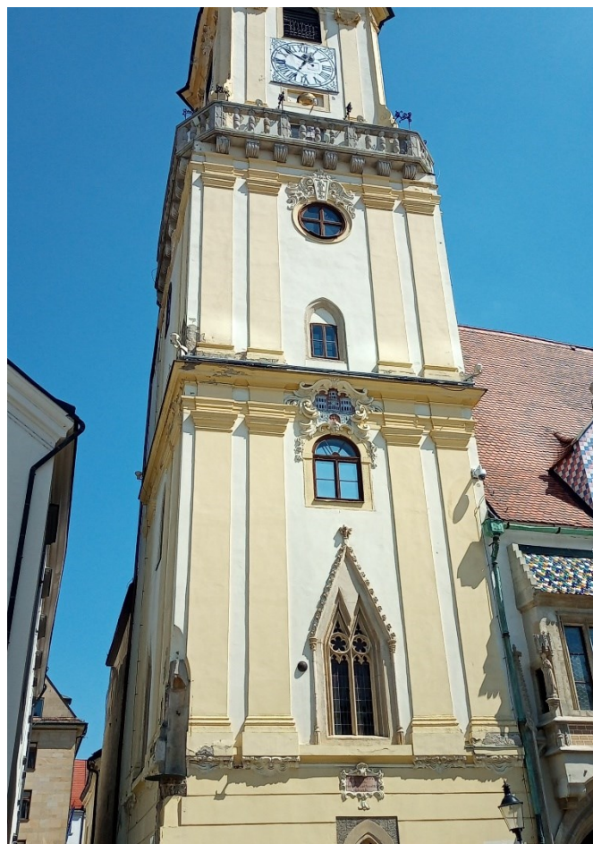
Fig. 15. The western facade of the tower with various presentations. The first floor – a late medieval double window, then a richly-decorated Baroque window, above the ledge a curvilinear medieval window and a Baroque elliptical window. (Photo: Author, 2023)
