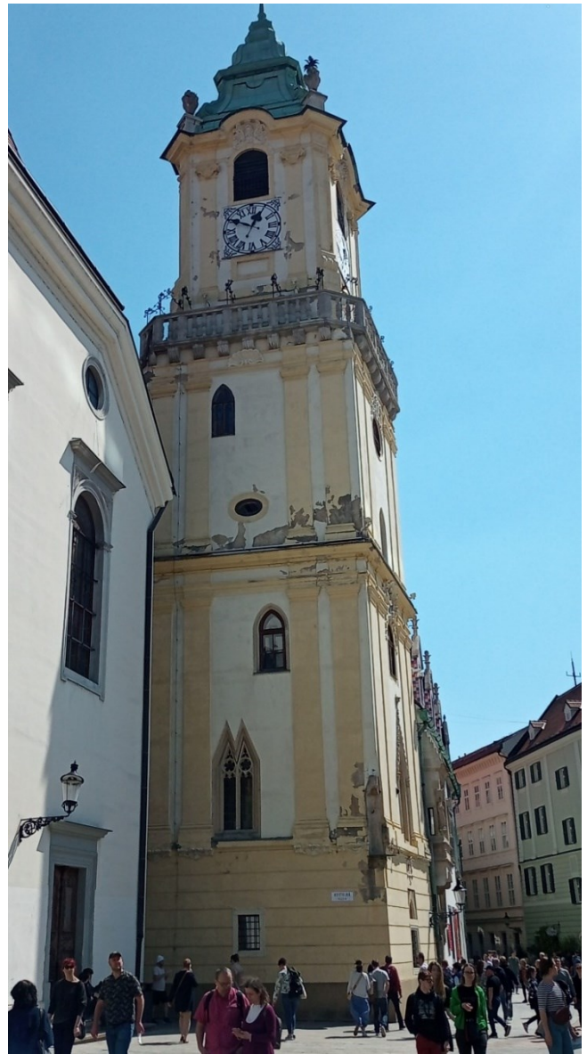
Fig. 17. The northern facade of the tower with various presentations. A Renaissance window on the ground floor, a late medieval double window on the first floor, then a curvilinear medieval window with stone framework, above the ledge a Baroque elliptical window and curvilinear medieval one. (Photo: Author, 2023)
