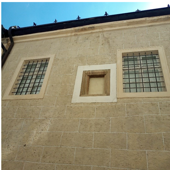
Fig. 22. Detail of the eastern part with two early Baroque windows and a medieval window (as niche). The surface is decorated with medieval network. (Photo: Author, 2023)
