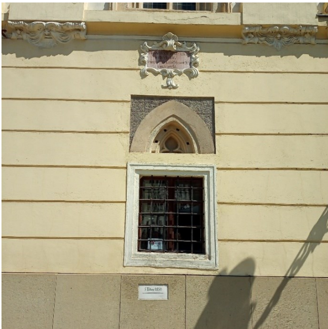
Fig. 16. Detail of the window on the ground floor – a curvilinear medieval form is presented analytically above a more recent window. (Photo: Author, 2023)
