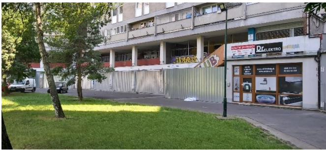
Fig. 4. Pentagon's parterre covered with metal sheets. (Photo: Šimkovičová, 2023)
