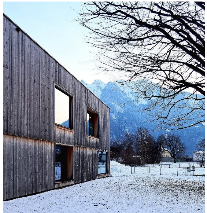
Fig. 15. A view of a ventilated facade that has naturally changed to a grey shade due to weather exposure. (Photo: Jakub Hanták, 2023)
