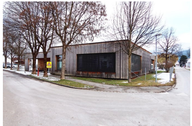
Fig. 14. The extension of the kindergarten building with a wooden cladding in Im Grisseler Street in the city of Feldkirch. (Photo: Jakub Hanták, 2023)
