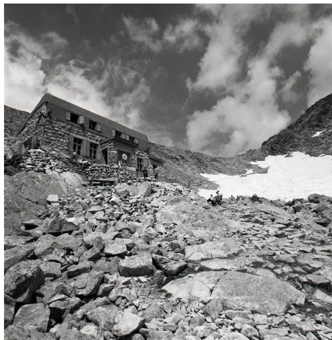
Fig. 10. Small intervention concerning Chata pod Rysmi in the form of sheathed superstructure. The façade remained without change, blending into the surrounding environment. (Source: TASR, 1986)
