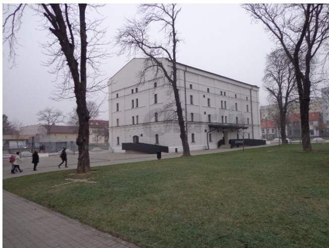
Fig. 25. Kulturpark in Košice, Slovakia: The Steelpark Museum building. (Photo: Filová, 2020)
