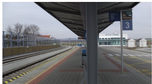
Fig. 1. Integrated passenger transport terminal in Moldava nad Bodvou mesto, Slovakia
