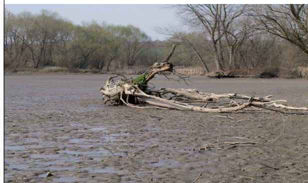
Figure 2: Reservoir filled by sediments. Photo: Jurik, 2017
