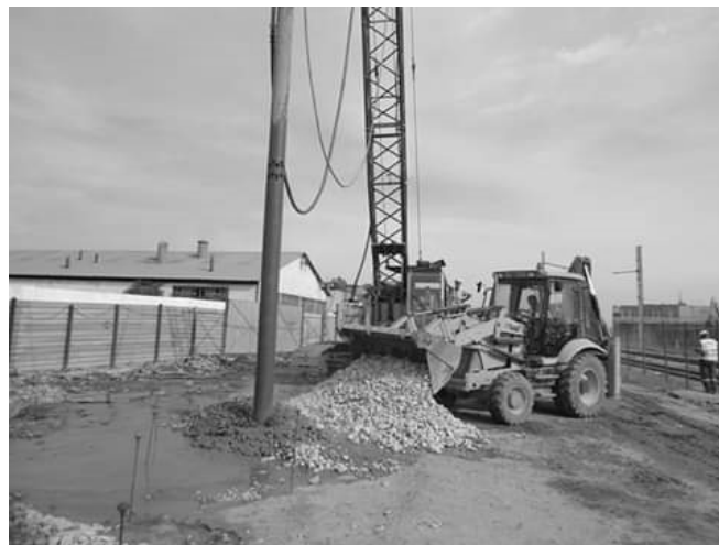
Figure 1: Realization of a wet stone column
