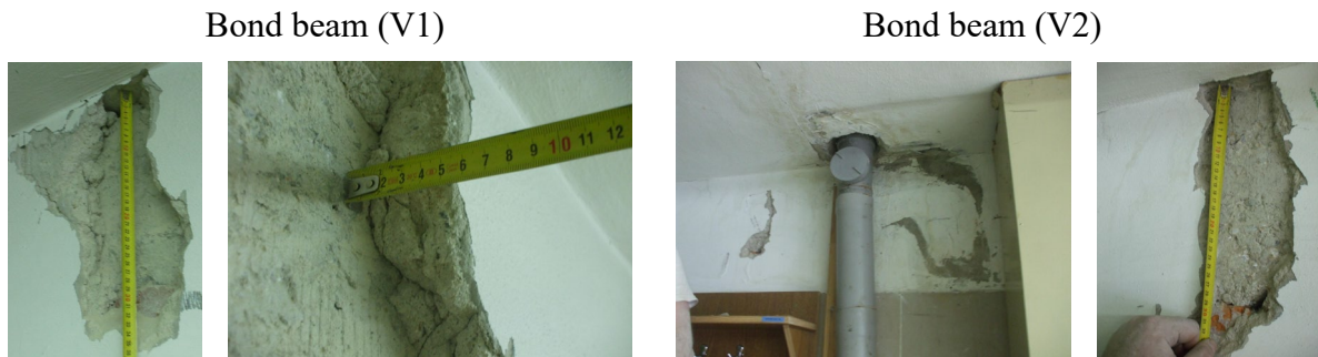
Figure 7: View of the reinforced concrete bond beam (V1) and (V2) height of bond beam (V1) is 28.5 cm, plaster thickness 5 to 5.5 cm height of bond beam (V2) is 29 cm, plaster thickness 2 cm
