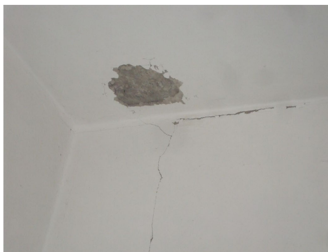
Figure 6: View of the precast concrete ceiling panel (PZD 5/475) in room 2103
