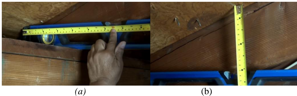
Figure 2: Measuring of the roof span (a), and roof rise (b)
