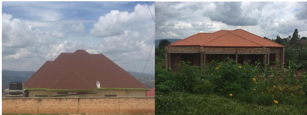
Figure 3: Residential Houses with different roof slopes
