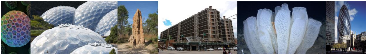
Figure 12: The Eden Project: The Biomes, Cornwall, UK, Grimshaw Architects – mimic structure of pollen seed; Figure 13: The Eastgate Centre, Harare, Zimbabwe, Mick Pearce – mimic cooling mechanism of a termite mound; Figure 14: 30 St Mary Axe Tower, London UK, Foster+Partners – mimic shape and lattice structure of a Venus' flower basket
