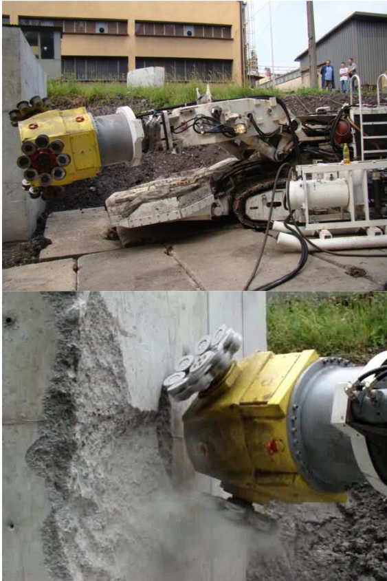
Fig.21. The new generation mining head with disc tools during field tests
