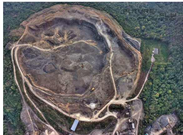
Fig. 12. Aerial survey of the open pit mine Vehec.
