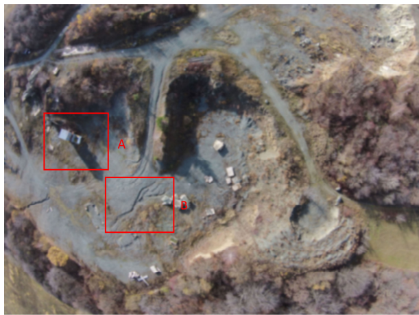
Fig. 15. Photos taken without the enhanced camera gimbal stabilization (A – building, B – grooved terrain).
