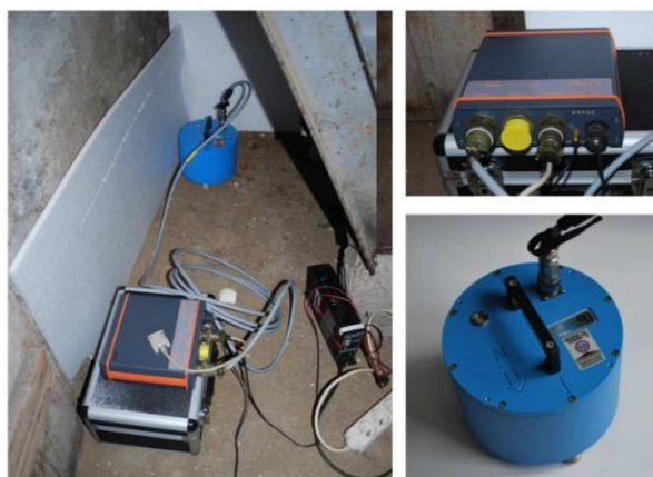
Fig. 2. Apparatus GAIA Q with seismometer Lennartz LE-3D/5s is installed in the cellar of a small masonry building at a depth of approximately 2 meters below the surface.
