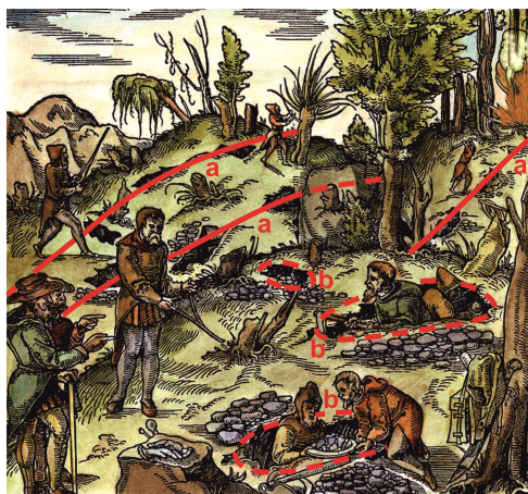
Fig. 3. Digging of exploration pits in the first half of the 16th century by G. Agricola (Agricola, 1556). Line grouping of pingens to pingens rows (a) and sheet layout of pingens into the pingens field (b).
