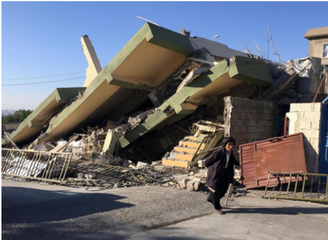
Fig. 1. A man walks past a collapsed building in Dabandikhan in Sulaimaniya Governorate, Iraq. (Photo by Ako Rasheed, Reuters; Received from http://www.interaksyon.com/toll-from-iran-iraq-quake-breaches-450/ ).
