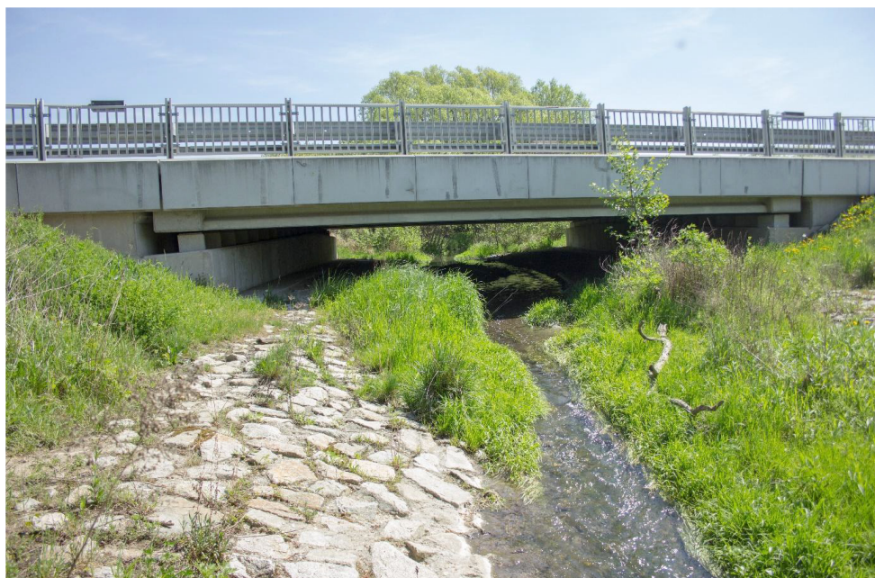
Fig. 6. The most used underpass (P31) in the solved area (photo: Novota, 2017).
