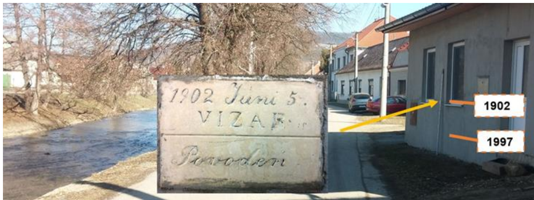
Fig. 6. Location of the flood mark from June 5, 1902 in Sobotište, level of flood in 1902 and 1997.
