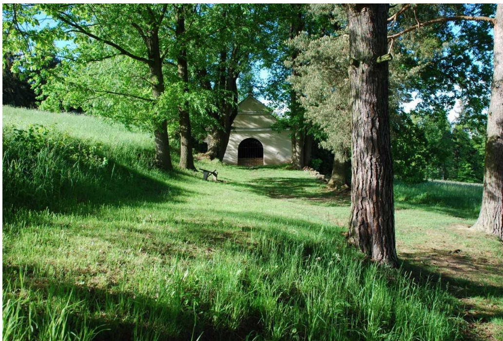
Fig. 4: Chapel called Deserted village (Gethsemane yard) built in 1691, renewed in the years 1778 and 1795 and classicist rebuilt in 1810 (Photo: Kupka 2013)
