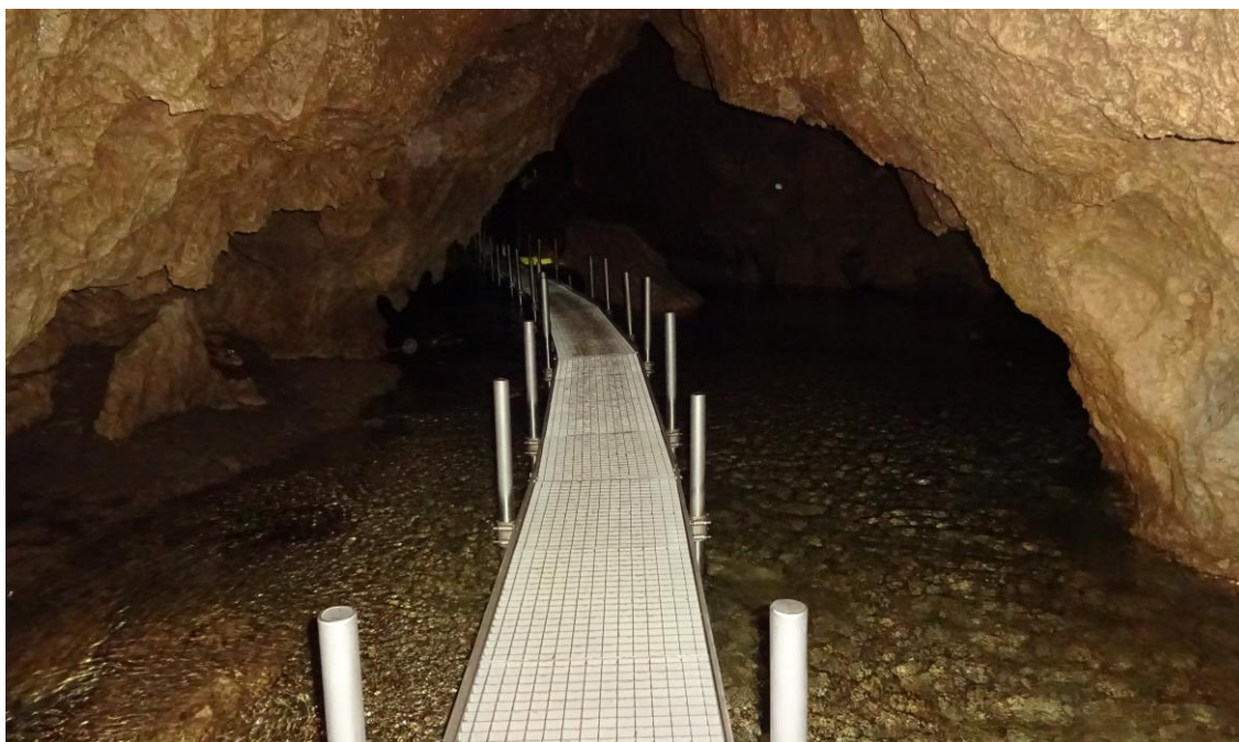
Fig. 4 Steel footpath over the underground river
