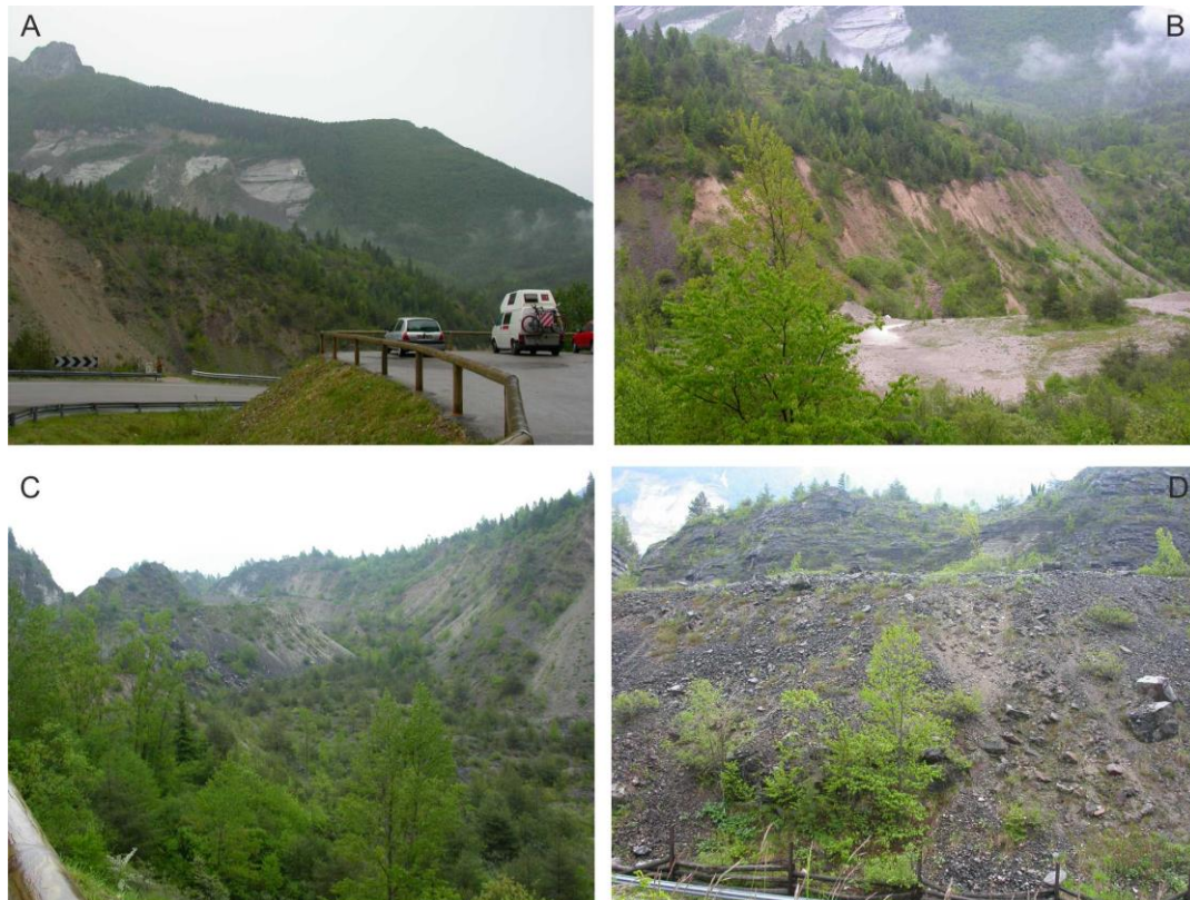
Fig. 8 Various packages of colluvial material at the valley bottom visible along the road from the Vajont Dam to Casso. Note brecciated marls of the Scaglia Rossa Formation (B) and rolled package of the Sowerzene Formation (D); total thickness of colluvial sediments (not visible on photographs) is estimated at around 250–300 m. Photos by: K. Bqk
