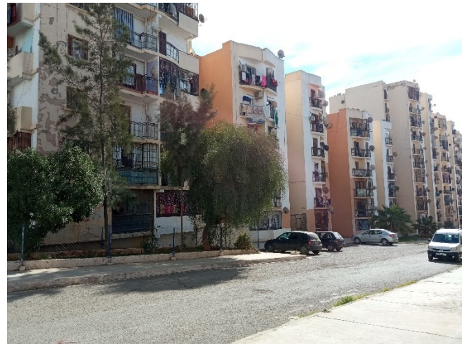
Fig. 3. View of the rear façade. (Source: Authors, 2023)
