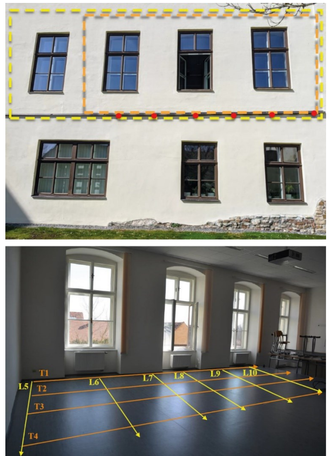
Fig. 3. Room 1.18 (yellow) and measurement area (orange). The red dots show the initial positions of the longitudinal (L) profiles, which were positioned according to the central axis of the windows. (top) Orientation marking of the square network of longitudinal (L) and transverse profiles (T) in room 1.18. (Author: Válek, 2021)
