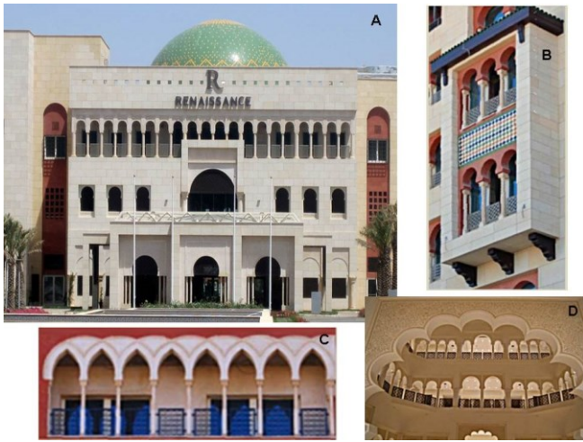
Fig. 11. The Marriott hotel façade. A) The main façade of the Marriott hotel; B) View of a moucharabieh supported by three brackets.; C) Details of an arched balcony; D) A poly-lobed arch with an arabesque frame. (Photos: Boulbene, 2012)
