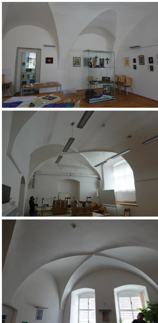
Fig. 1. Barrel vaults with lunettes under room 1.11 (top), cross vaults under room 1.11 and room 1.12 (middle), barrel and cross vaults under rooms 1.17 and 1.18 (bottom). (Photo: Válek, 2021)
