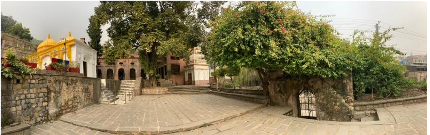
Fig. 18. Saidpur's main node with heritage temples and Dharamsala, with old entrance gate. (Source: Ramsha Nazir Malik)
