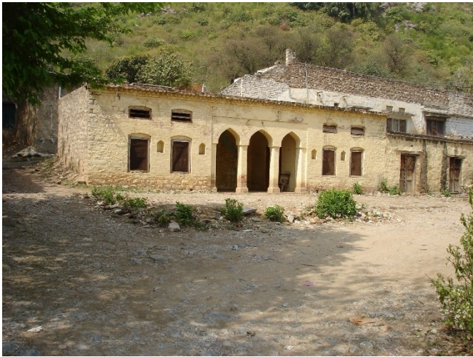
Fig. 29. Old Haveli before renovation. (Photo: CDA)
