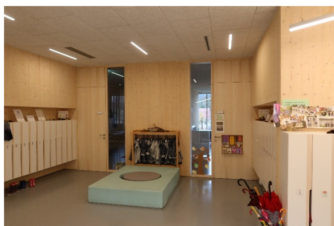
Fig. 12. Hallway space and a view of the playroom with CLT load-bearing panels with a fine finish. (Photo: Jakub Hanták, 2021)
