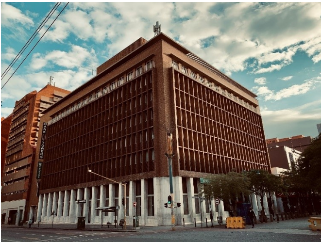
Fig. 6.1. The Nedbank building in context. The facade showcases the deep set and sun shy window motifs. (Photo: Cornelius van der Westhuizen, 2022)
