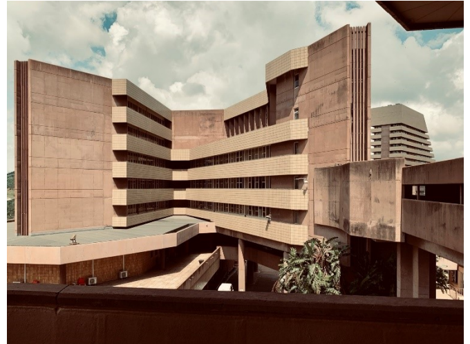
Fig. 13.3. The sculptural and refined massing of the buildings; also note the deep eaves and covered walkways. (Photo: Cornelius van der Westhuizen, 2022)
