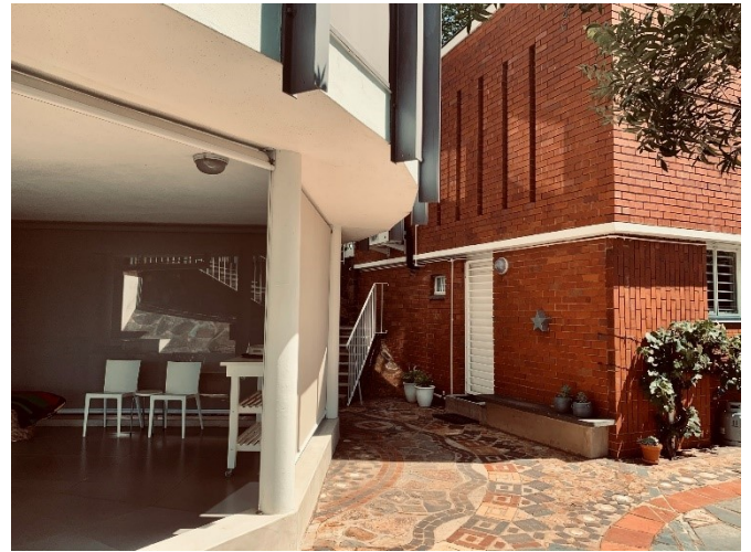
Fig. 9.2. The Round House exterior detail, the pilotis raise the building from the ground and create an open but covered verandah. (Photo: Cornelius van der Westhuizen, 2022)
