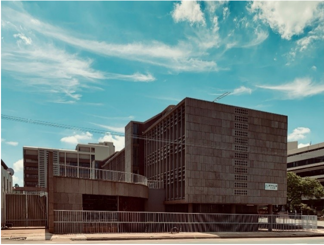
Fig. 7.2. Street level interface and solar shading devices. (Photo: Cornelius van der Westhuizen, 2022)
