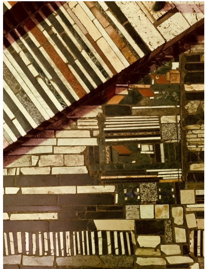
Fig. 8.3. Floor pattern detail. Offcuts from granite tombstones were meticulously laid in patterns. (Photo: Cornelius van der Westhuizen, 2022)
