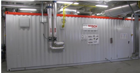
Figure 3 Container with cogeneration unit
